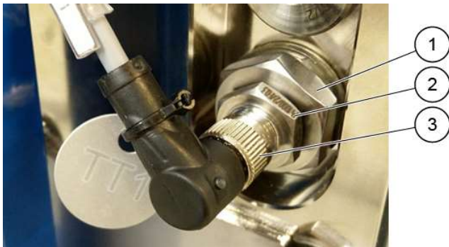
Figure 41. Temperature sensor mounted into temperature sensor pocket. Sensor location may vary depending on cooling station model.
